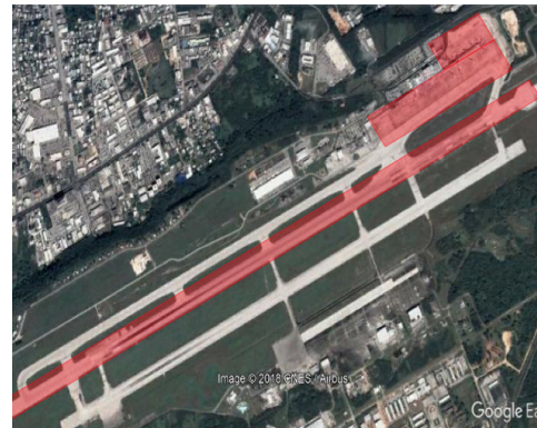
Runway 6L Rehabilitation And Airport Aprons & Taxiway Rehabilitation
