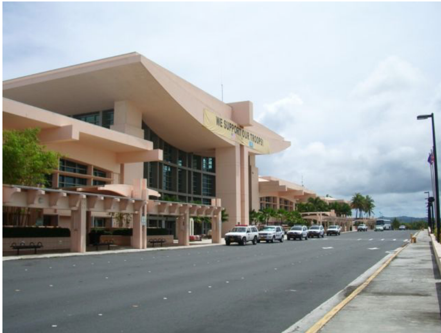
Figure 4.3: View of Passenger Terminal front and the departures drop off roadway
