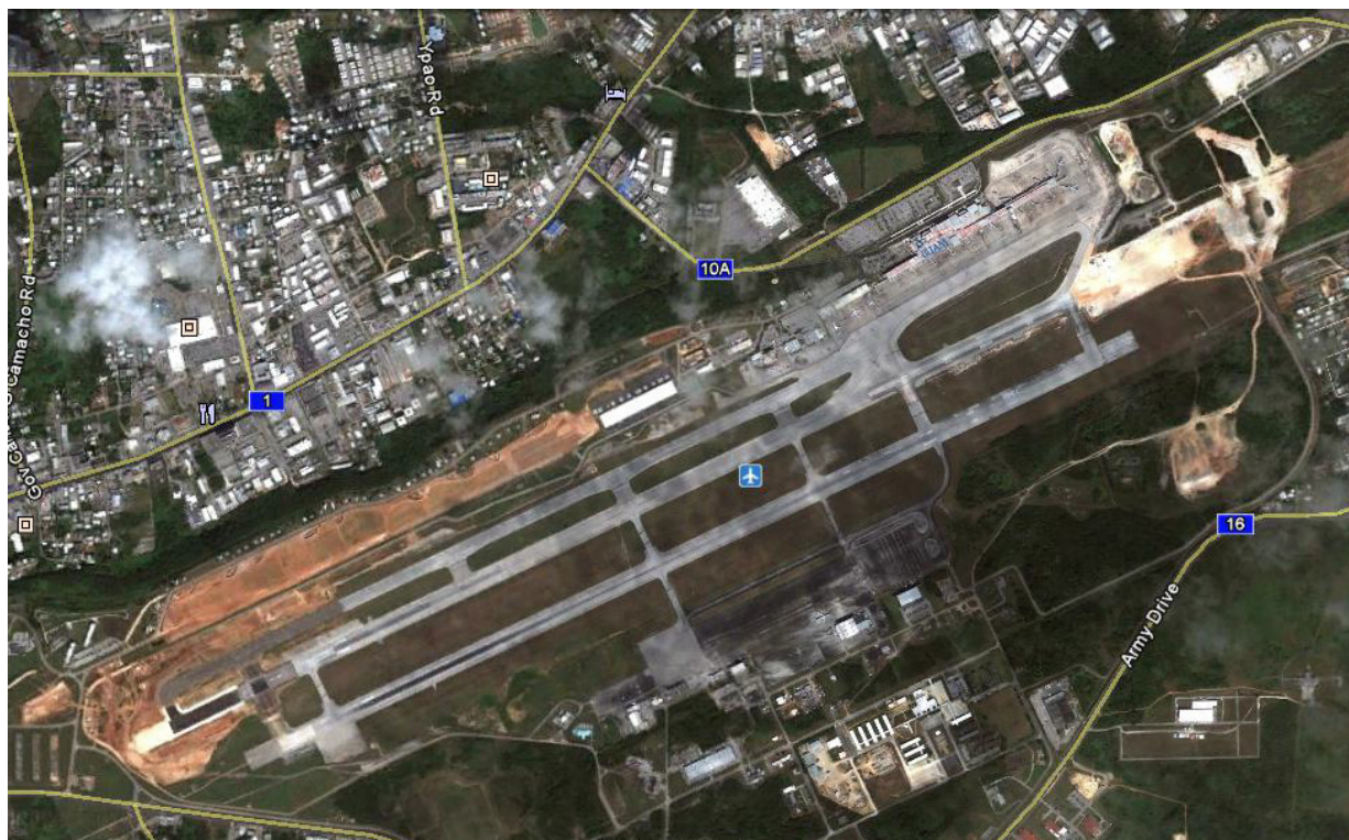
Figure 4.69: Aerial Photograph of the Airport and Surrounding Environs
