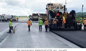
RUNWAY PROJECT 6L/24R Asphalt Laying on Primary Runway Completion Target: Nov. 2021
