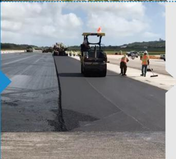
Phase I of the Rehabiliation of RWY 6L/24R is about complete. Asphalt is laid on Taxiway J in the photo. Phase II is expected to commence soon, addressing re-habilitation needs and striping work between Taxiway C and D.
