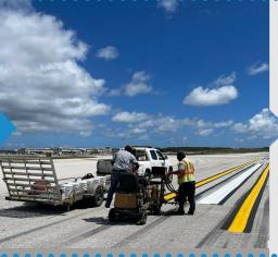
Runway 6R/24L centerlines and lead lines are marked professionally by the Airport's Properties & Facilities painting crew. Runway markings are important in enabling the airplane to navigate and avoid incursion on the runway.
