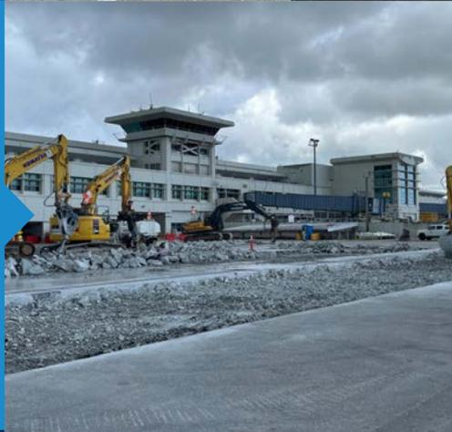
Rehabilitation of the Apron and Taxiway is well underway at Gate 10 of the main terminal building. This project, which broke ground in March this year, will address and resolve any reported distresses along the aircraft parking aprons and taxiways. Upon completion of this project, the north apron pavement and taxiway will be re-vised, extending the pavement life for years to come.
