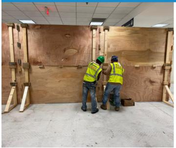
Floor prep work and installation of hoarding walls have begun in anticipation of the installation of new flooring in the U.S. Customs & Border Protection (USCBP) Hall and in the Baggage Claim Area. Carpet in both areas were removed as a result of water damage caused by Typhoon Mawar in May 2023 and will be replaced with terrazzo floors. Contractors, seen in the photo above, install hoarding walls
