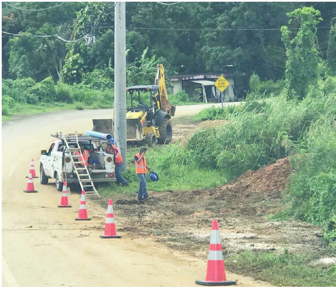
DIGGING IN: A Guam Waterworks Authority backhoe digs into an area along Casimir Street in Mongmong on Saturday morning to uncover a water pipe that has broken. It's the third break in the line this week, residents say. Photos by Oyaol Ngirairikl/The Guam Daily Post
