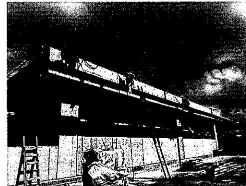
Main Roof Precast Panel Support Welding
