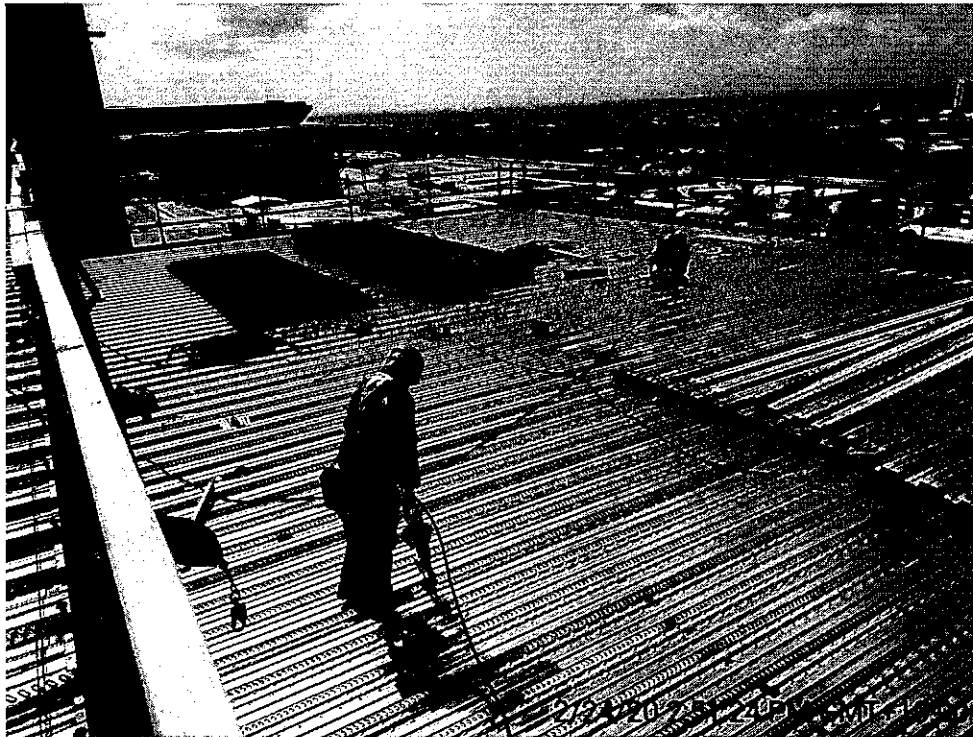
Placement of Metal Deck Wire Mesh
