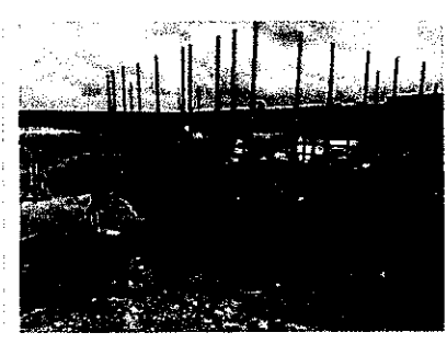
STORM DRAIN LINE JUNCTION BOX 31' x 17' x 8'
