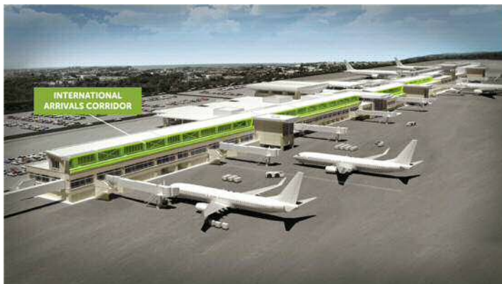
The IAC, highlighted in green, sits atop the current terminal, and will provide direct routing of arriving passengers to passenger inspection points when complete.
